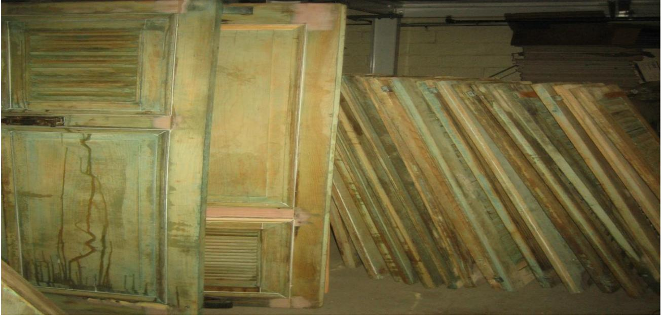
Most had damage but many were beyond repair. We contracted Timberlane Shutters of Pa. to make replicas of the shutters and the associated hardware. **(Picture #9 New Shutters)** This was so that the entire building would have matched shutters and hardware everywhere on the building.
