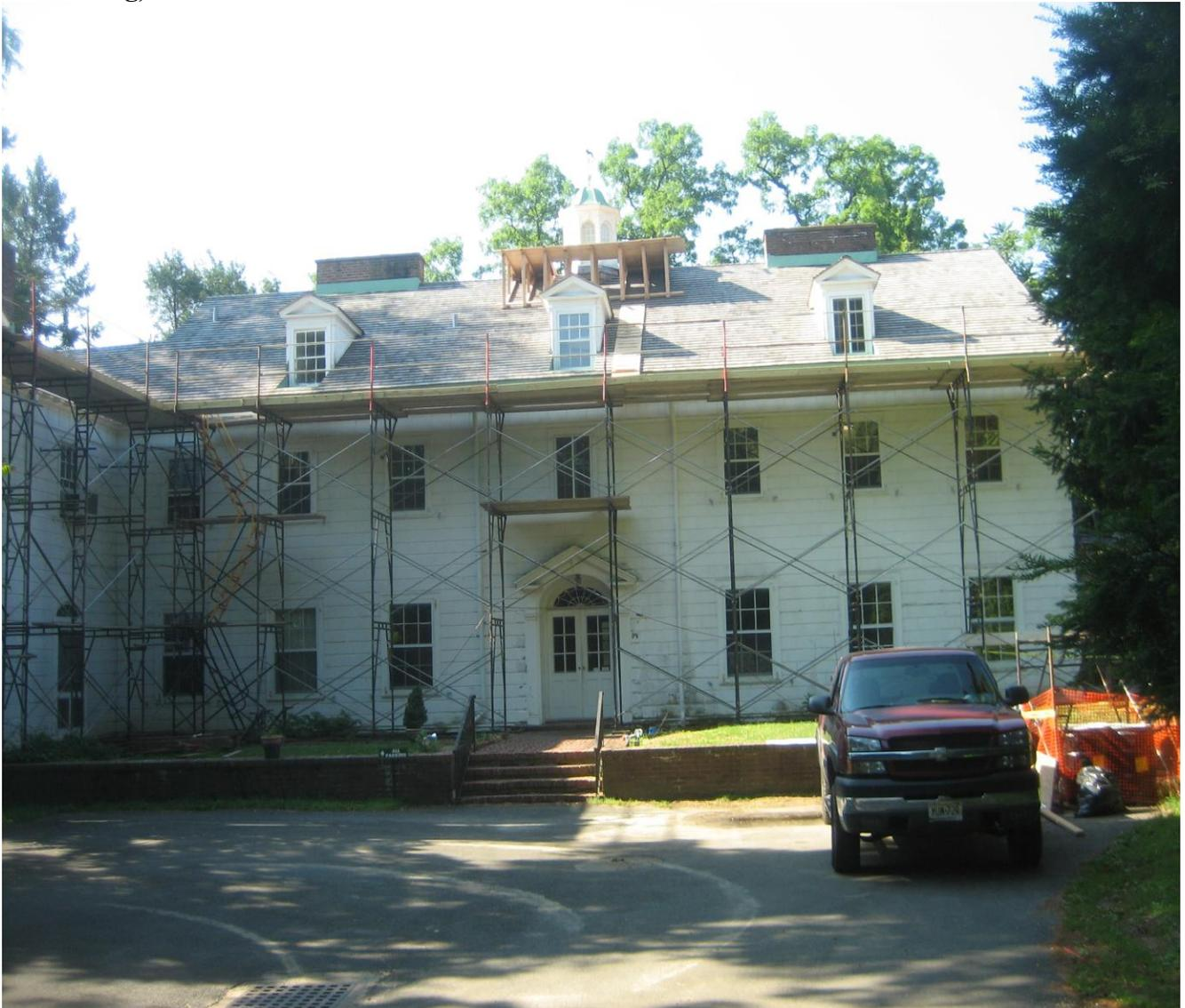
It was installed with the required safety railing system and numerous posted signs. The scaffolding was inspected daily by site supervisors to ensure it was safe to work on. Additionally, after the scaffolding was erected the scaffold planks had to be individually secured with wire to the frames due to an impending hurricane (Hurricane Earl) that was forecasted to hit the area. Fortunately, the hurricane moved further out to sea and was primarily a rain event.
