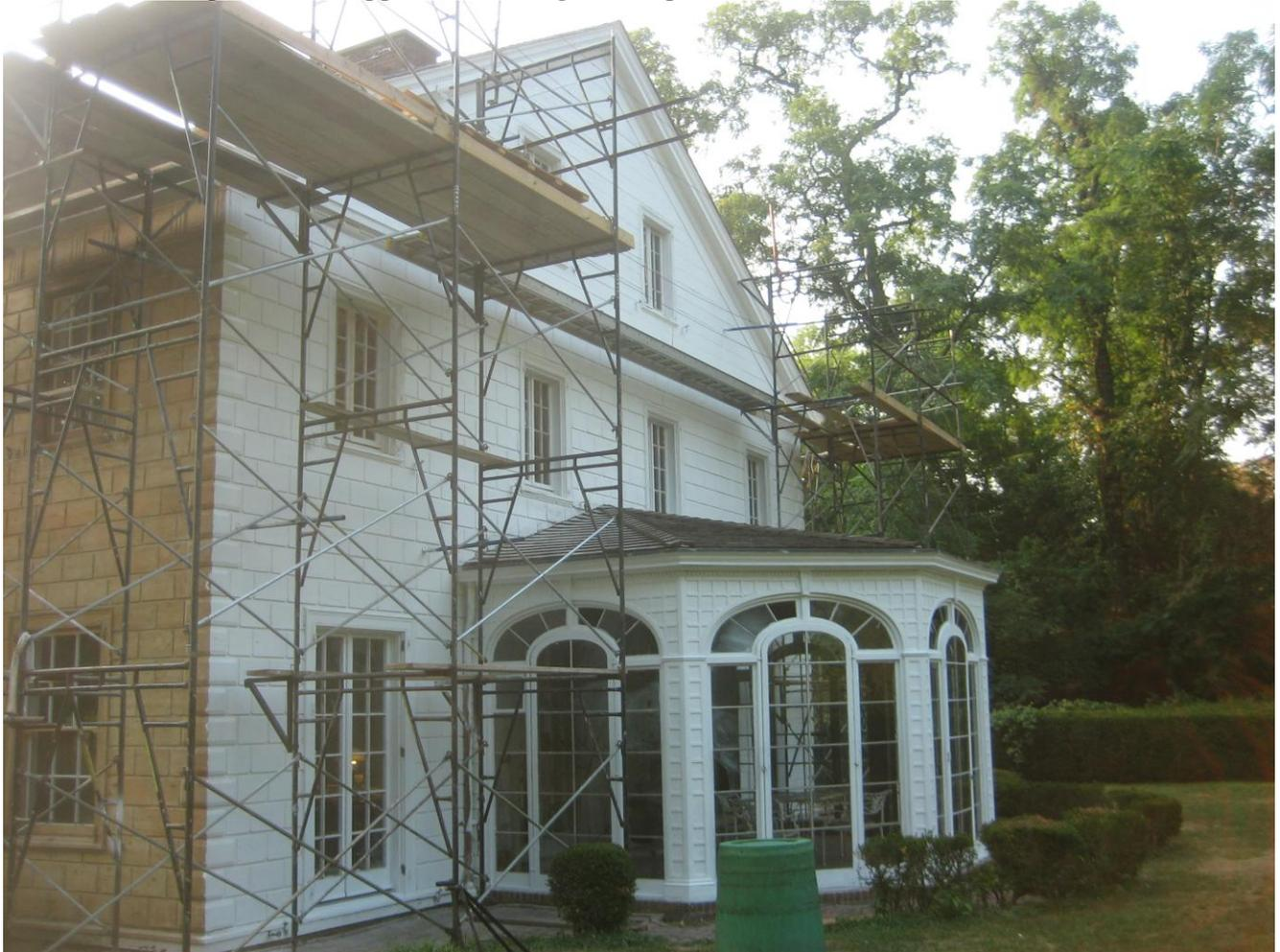
This was completed and approved by the inspector. We then moved on to applying the finish coat of Sherwin Williams A-100 100% Acrylic Latex, Flat Finish Topcoat, which was also sprayed on the exterior of the Hall. With great hiding capabilities and color retention A-100 Flat is Sherwin Williams best quality exterior flat finish.
