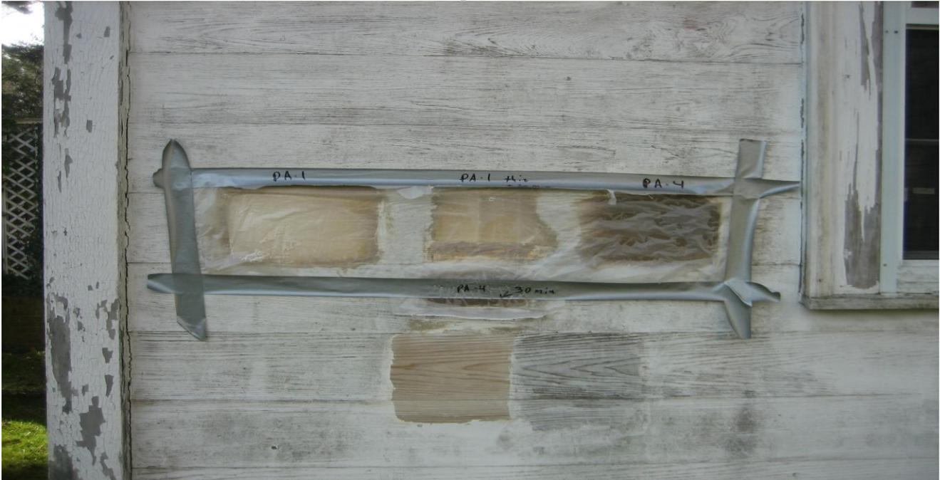
It took over 500 gallons of Peel Away 1 on over 11,000 square foot building to remove all of the old layers of paint. The product was sprayed on and removed by hand. All hazardous material generated from the preparation phase of this project, was removed from the site in accordance with all local, state and federal laws. **(Picture #5 Hazardous Material)**
