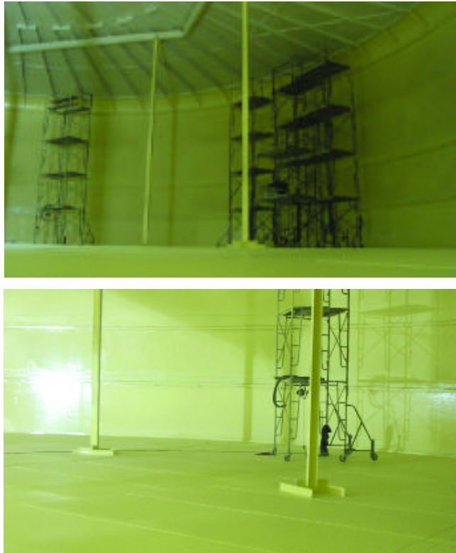
Tank nearing completion and return to service
